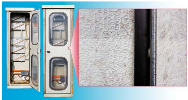
Figure 2: The gel coat of this GRP cabinet is still intact and there are no loose fibres, 40 years after installation at an oil refinery.
