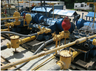
Pulsation dampeners (red and yellow cylinders) connected to the discharge manifolds of triplex mud pumps, with vibrator hoses attached.
